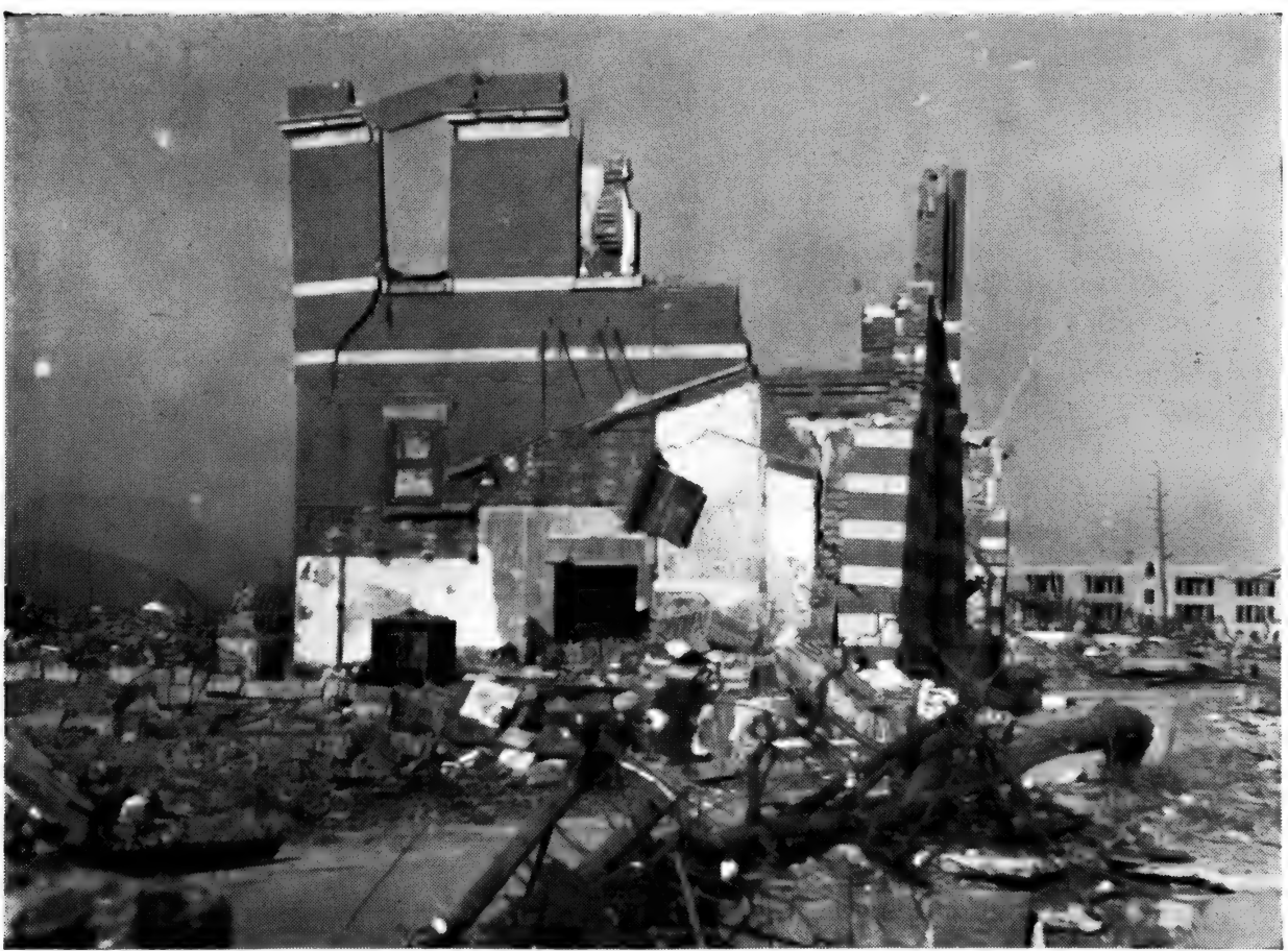
Photo No. 15. HIROSHIMA. Three storey bank building with load-bearing brick walls of strong construction and comparable with British standards. This degree of damage to such buildings extends to a radius of \frac{1}{2} mile from centre of damage. Compare with the behaviour of the reinforced concrete framed building in the background. See paragraph 38.
